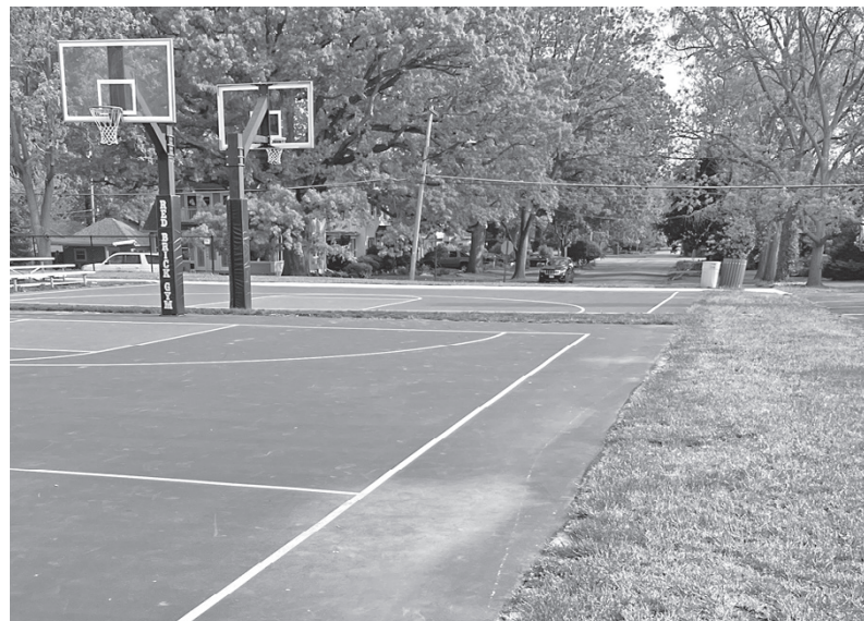
fencing will enclose the basketball court area adjacent to the parking lot.
