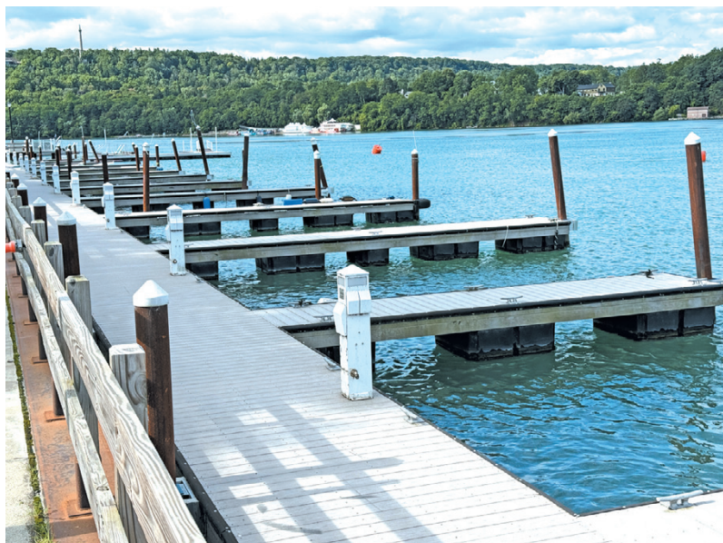
The Village of Lewiston Board is working toward finding a permanent solution to weather threats against the waterfront dock.
