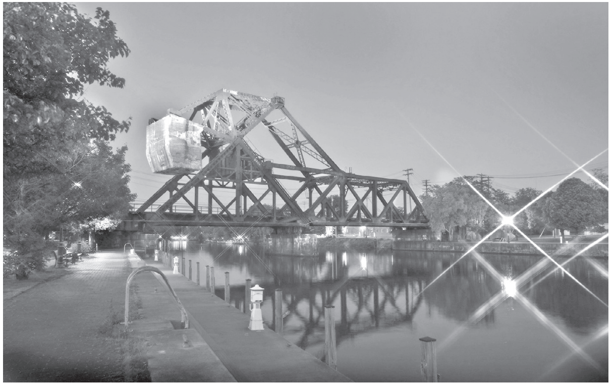
Iconic lighting for the CSX railroad bridge over the Erie Canal of the New York State Canal Corp. (Photo by Paul Pasquarello, for the New York Power Authority)
