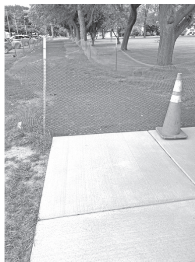
Uneven surfaces will be remedied before the bathrooms reopen.
